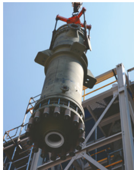
↑ Disassembly of a used DIABON heat exchanger
