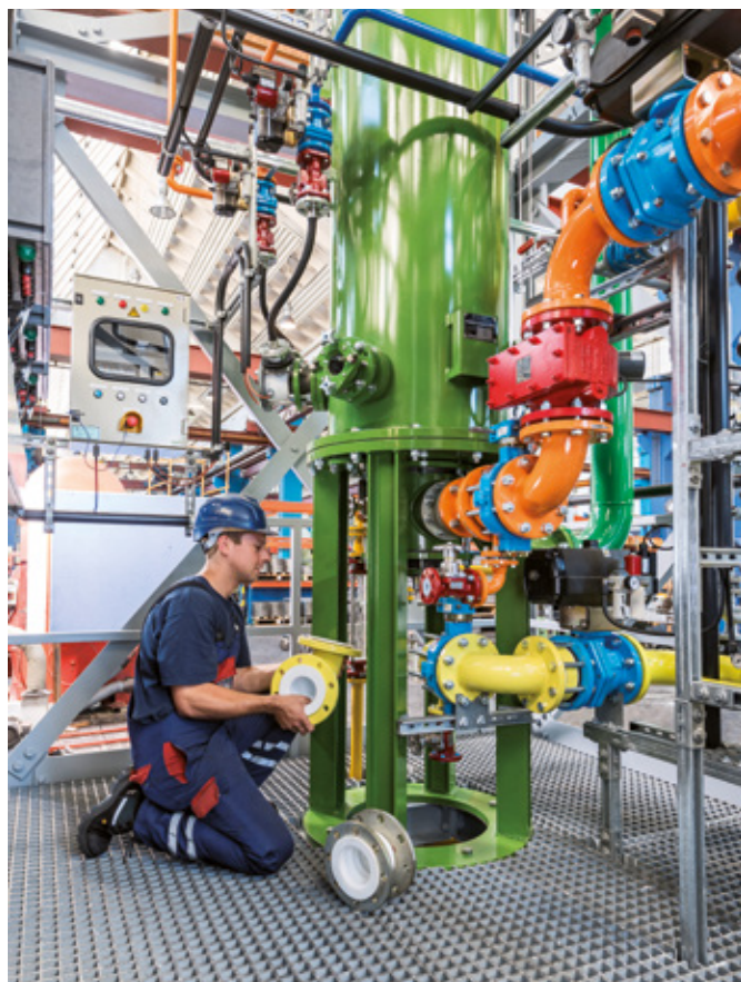
↑ Initial assembly of chlorine feed pipe at a HCl synthesis unit
