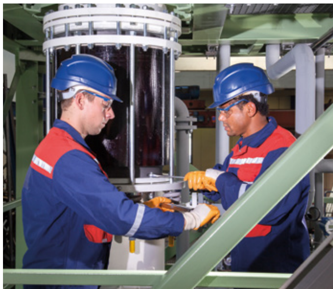
↑ Final inspection of a flange connection before start-up
